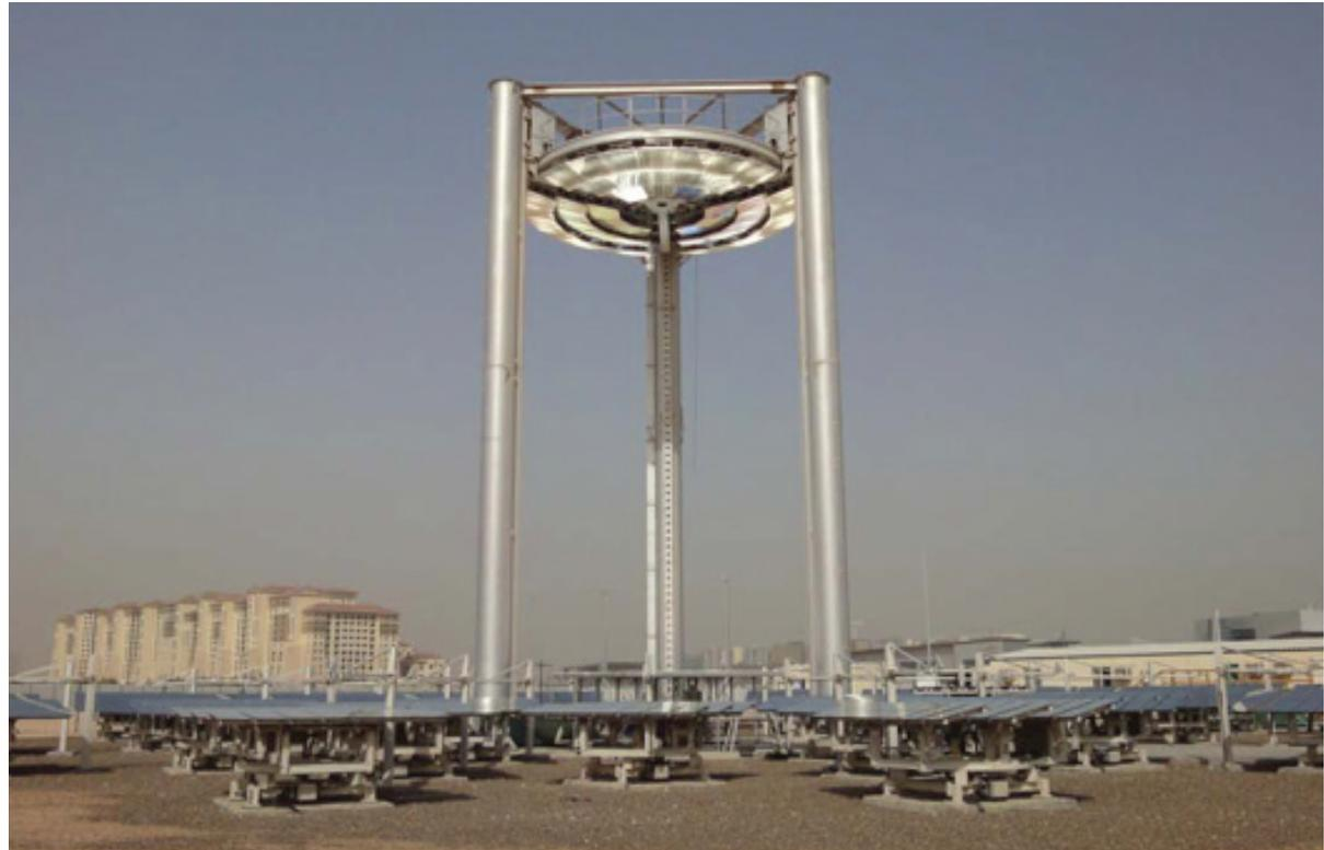
**Beam-down point-focus CSP heliostat array at Masdar**
