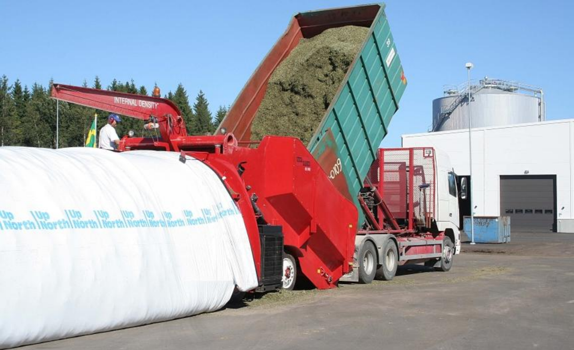
Västerås Biogas Plant, Sweden, Start up - 2005; Source: T. AlSeadi, Department of Bioenergy, SDU, Denmark
