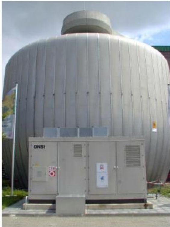
PC25C Fuel Cell in the WWTP Rodenkirchen
